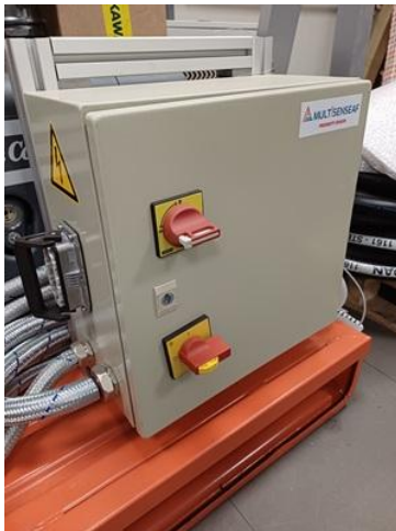
Figure 12. Blower electric box that manages the three-phase power supply for the air pump's on/off control
